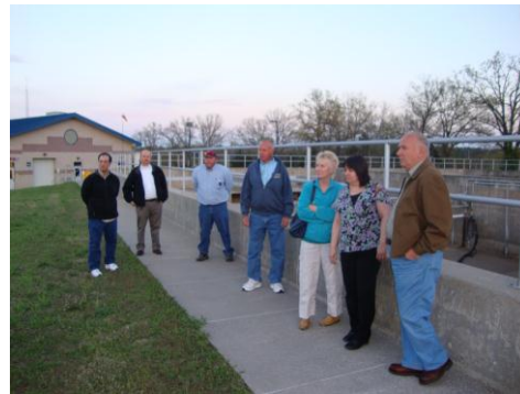
Visiting a city water treatment plant.
